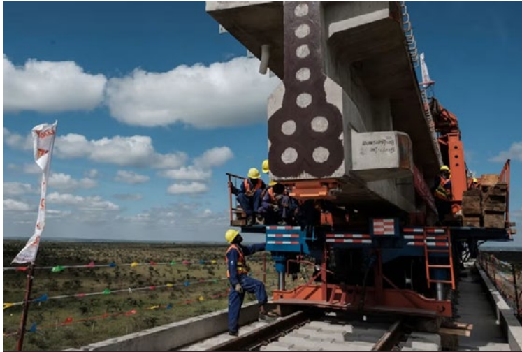
A railway project in Nairobi, Kenya, a signature project of China's Belt and Road Initiative. China's overseas investment has ranked in the top five of the world total for many years, and it has sought commercial success and geopolitical power—this is not worse than other capitalist countries, but neither is it better.
